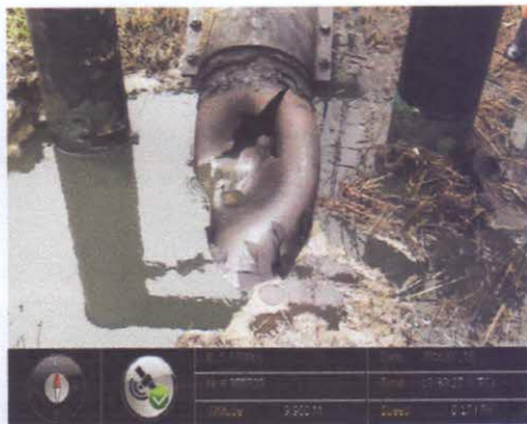
showing the blasted pipeline.
